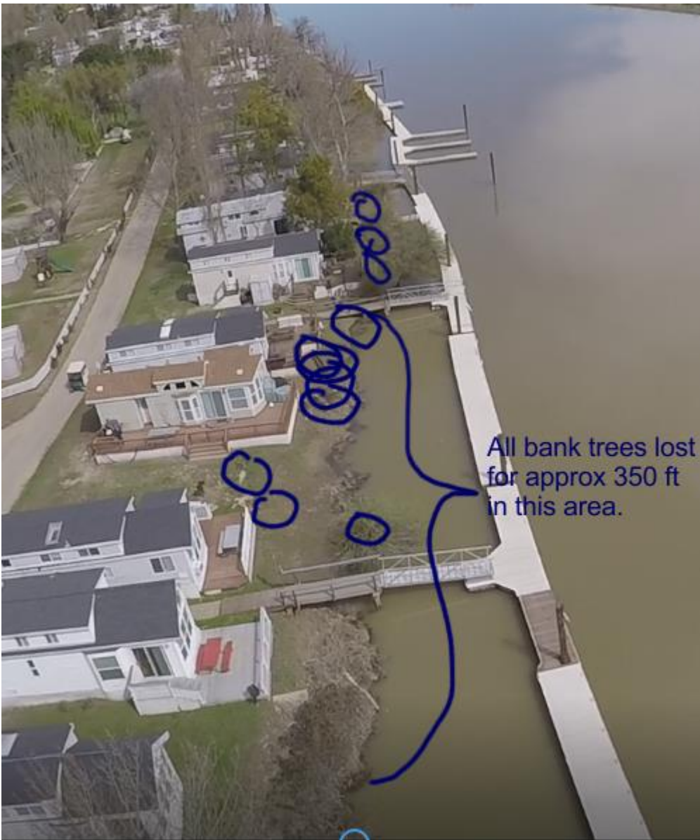
Above photo shows Snuggle Inns 9, 10, 11 and then the leaseholder park model RV cottages. Blue circles show the locations of trees that died 2016-2017 and fell, or had to be removed before falling.
